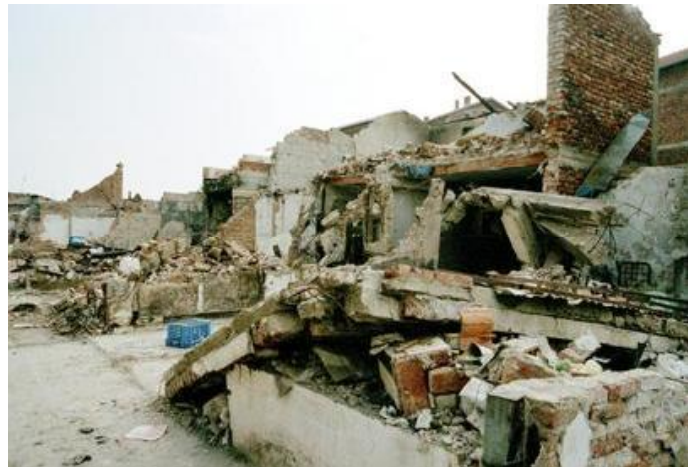
A section of the destruction in Pec, Kosovo. 14 Oct 1999. Photo taken by Milton Grant. http://downloads.unmultimedia.org/photo/medium/789/78978.jpg
